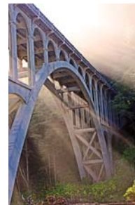
Hwy 1 Bridge John McCormack
